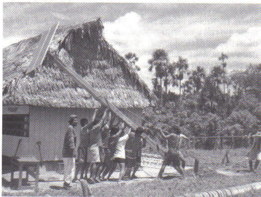
A solar panel is erected to power the telecommunications system
